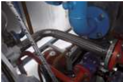
Stainless steel hose in a combined heat and power plant with 90° bend with swivel flanges on one side and welding ends at the other side.
