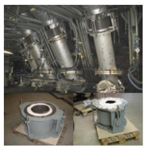
Penstock (gas nozzle) expansion joint for use in blast furnaces and very high operating temperatures
